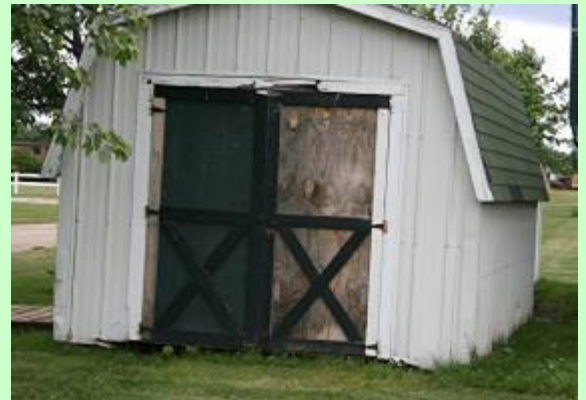
Scrape and paint the doors of the horse storage building
