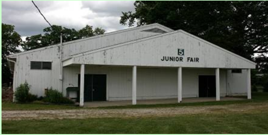
Junior Fair Building Scrape and paint West End
