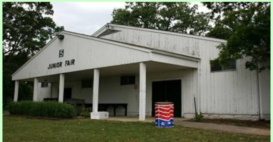
Junior Fair Building Scrape and paint East End
