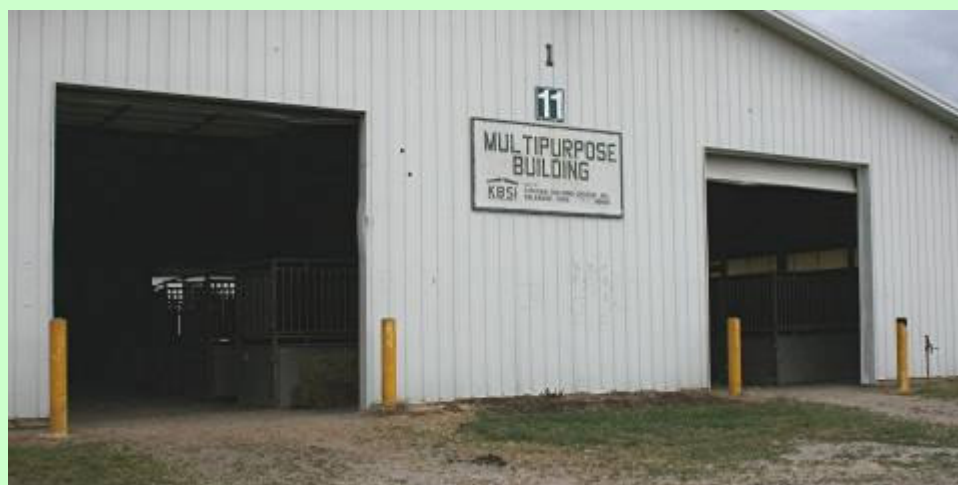
West Side Steer barn
