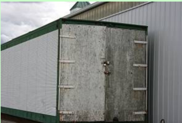
Scrape and paint the doors of the steer storage building
