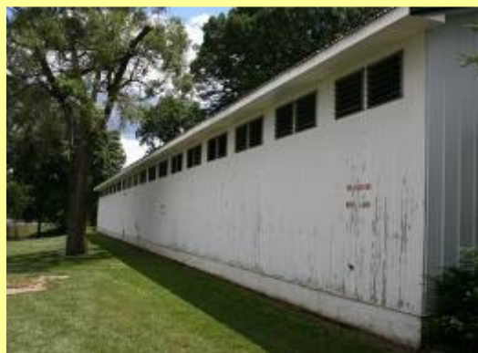
Scrape and paint North Side
