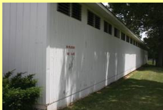
Scrape and paint South Side
