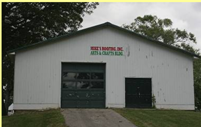
Scrape and paint East End
