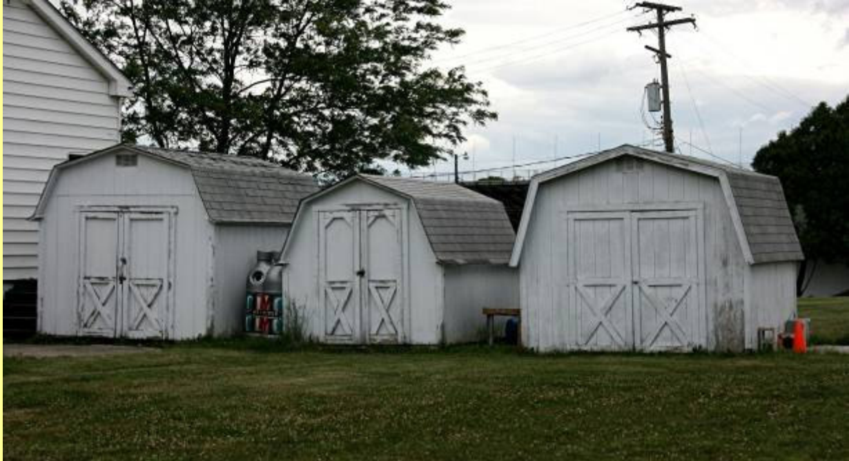
Scrape and paint building 4, 5, or 6 as numbered left to right
