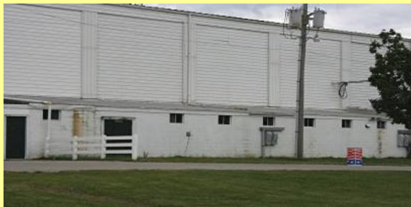
South Side scrape & paint
