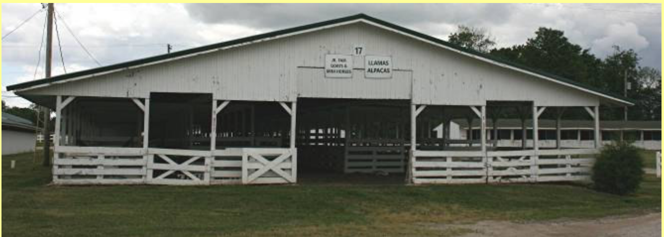
Scrape and paint East End
